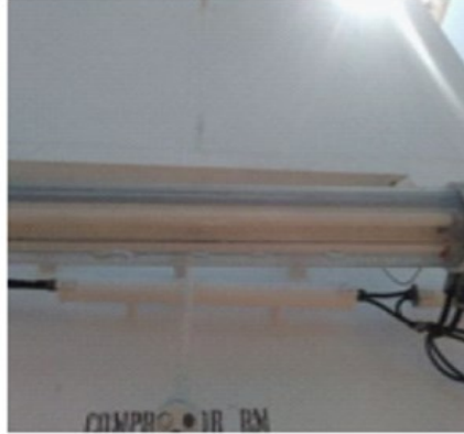
Standing Water in a Certified Safe Flameproof Light Enclosure Indicating Failed Ingress Protection
